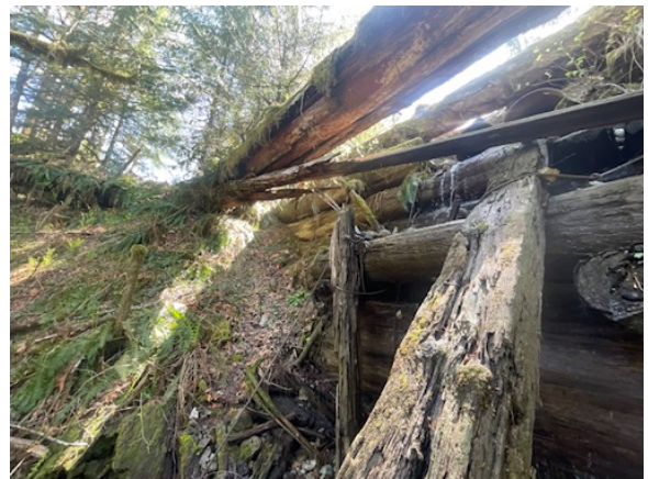
Outlet of drain pipes
